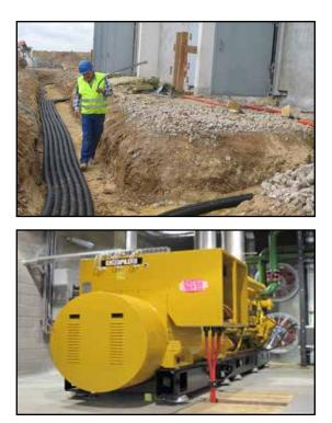
The feed & return line from tank to generator room runs into secondary ducts. Between 1 to 4 primary lines can be inserted into secondary ducts with diameters 3 1/2", 4 1/2" and 6". Both primary pipes and secondary ducts are laid in continuous runs, without buried inaccessible joints. At both ends the primary pipes are sealed with the secondary duct by means of flexible boots and special donuts. The boots are equipped with a valve for eventual continuous monitoring of the interstitial space.
