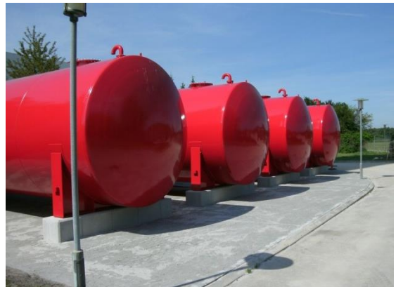
4 x 100 m 3 tanks diameter 2900 mm
