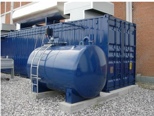
5 m 3 tank diameter 1600 mm
