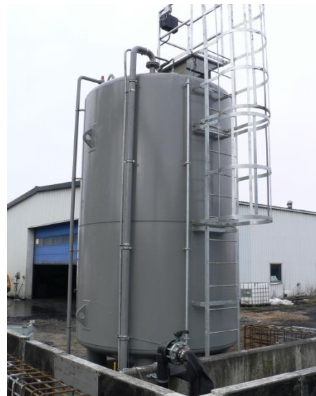
20 m 3 tank diameter Ø 2500 mm. With ladder and platform on top of tank, fill point to ground level.
