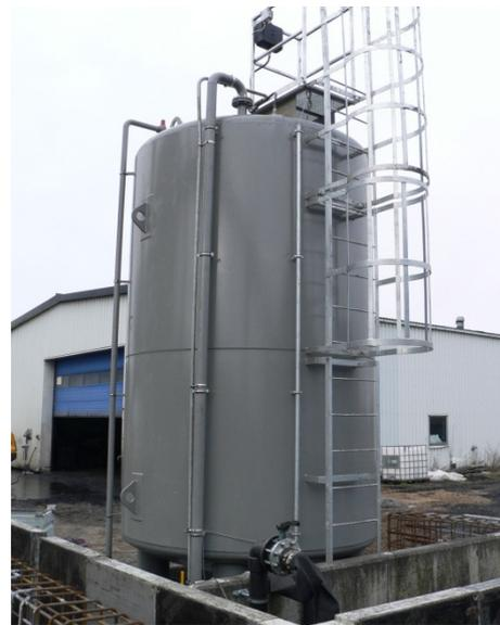
20 m<sup>3</sup> tank diameter på 2500 mm. With ladder and platform on top of tank, fill point to ground level, leak detection system etc.
