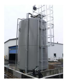
20 m³ tank diameter på 2500 mm. With ladder and platform on top of tank, fill point to ground level, leak detection system etc.
